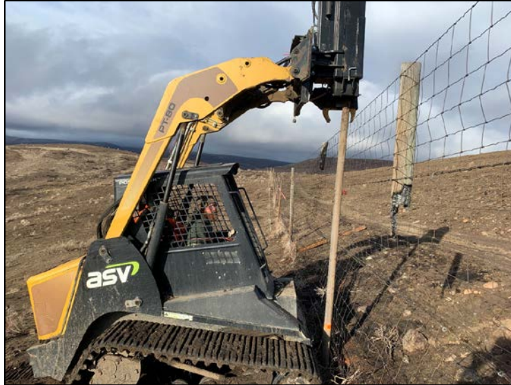
Natural Resources Technician Stultz driving metal sucker pipe along burnt section of the Bull Pasture elk fence
